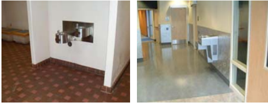
Alcove or wing wall removes the drinking fountain from the circulation path
